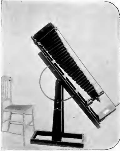
FIG. 13—Tilting Camera Stand in position for side window lighting.
